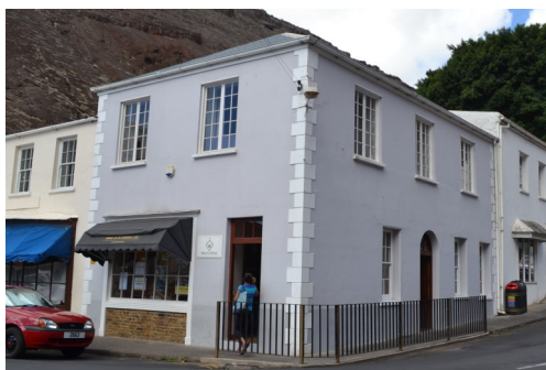
Main Branch, Market Street, Jamestown
